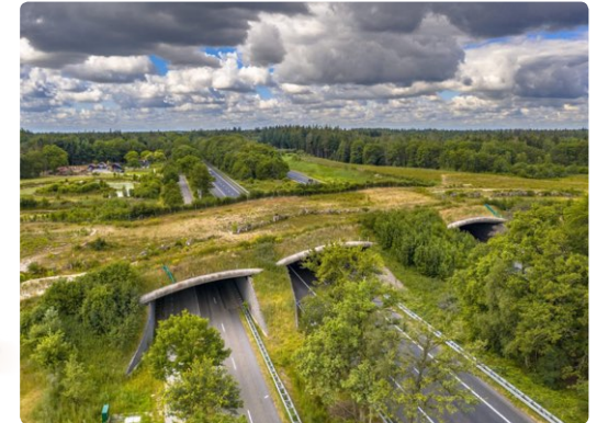
Wildlife overpass enabling wildlife to cross 3 highways at the same time © Centre for Large Land Conservation. https://largelandscapes.org/news/invest-act/
